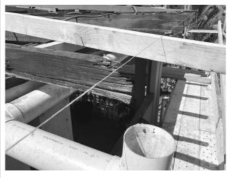
Rotten roof timbers once again. Entire front eaves also need replacing.
